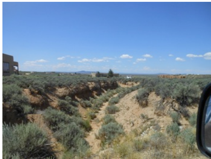
Treatment Plant Arroyo, Subdivision near Golf Course, note eroding banks
