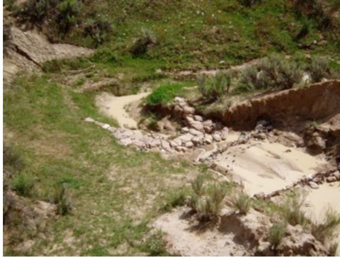
Hand-built cross vane in Cuba, NM
