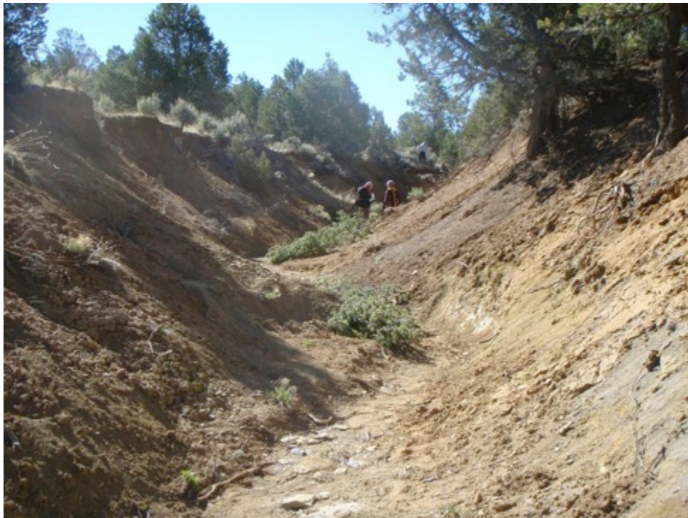
Pinon trees used to meander an arroyo and create floodplain.
