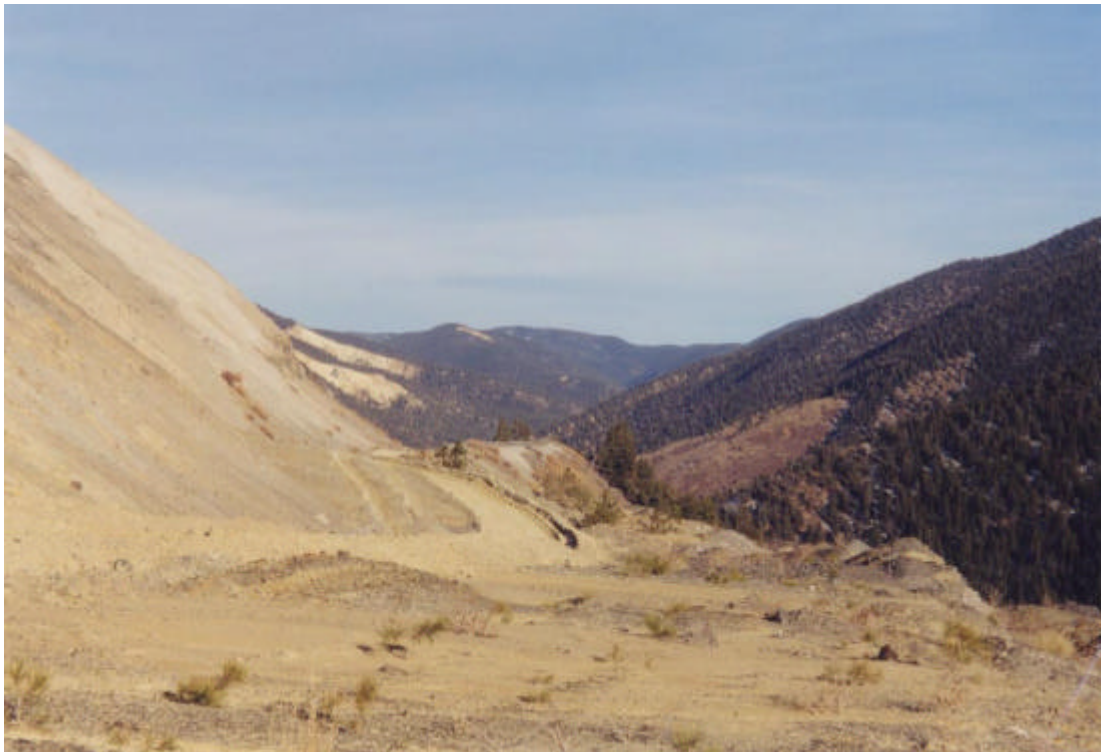
Picture 8. Waste Rock Dump (Middle) Bench (note stormwater control ditch and bench slump area).
