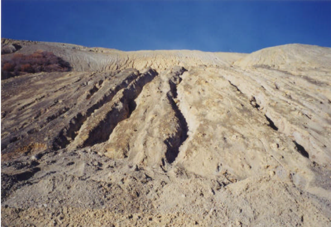
Picture 7. Waste Rock Dump (Middle) Erosion Gullies and Eroded Material.
