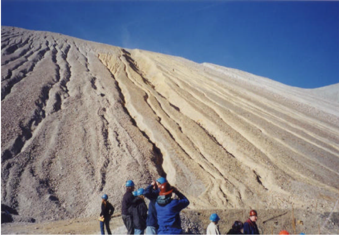
Picture 5. Waste Rock Dump (Spring/Sulphur Gulch) Erosion Gullies.
