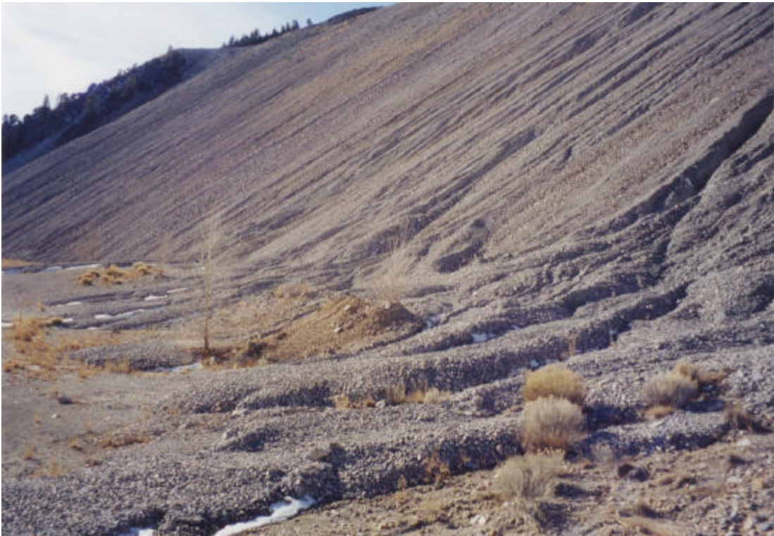
Picture 6. Waste Rock Dump (Spring/Sulphur Gulch) Eroded Material.
