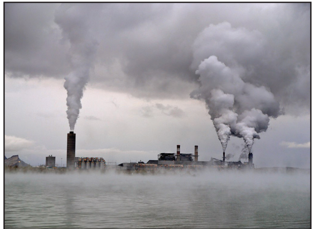
Four Corners Power Plant 167
