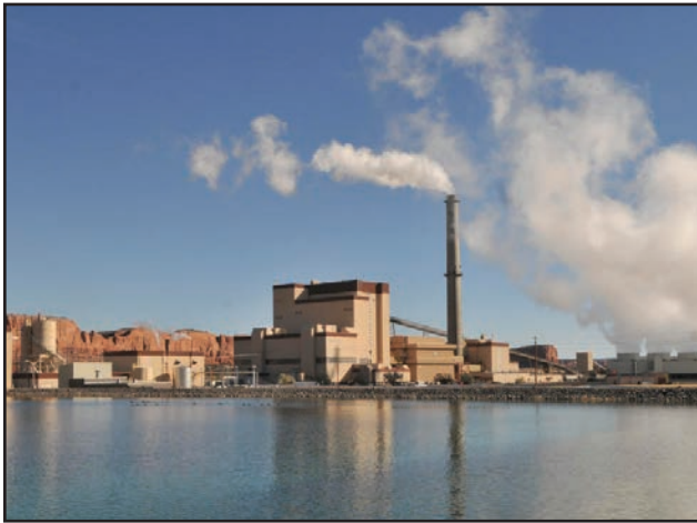
Escalante Generating Station 168
