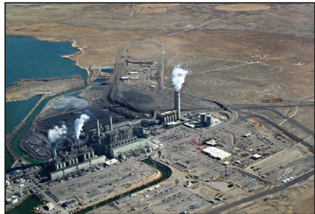
Four Corners Power Plant 238
