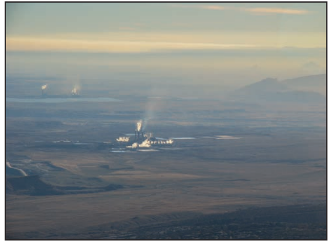
San Juan Generating Station with Four Corners Power Plant in the background 169
