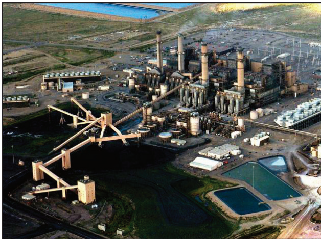
San Juan Generating Station 166
