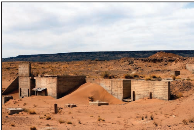
Abandoned uranium mine on the Navajo Nation 546
