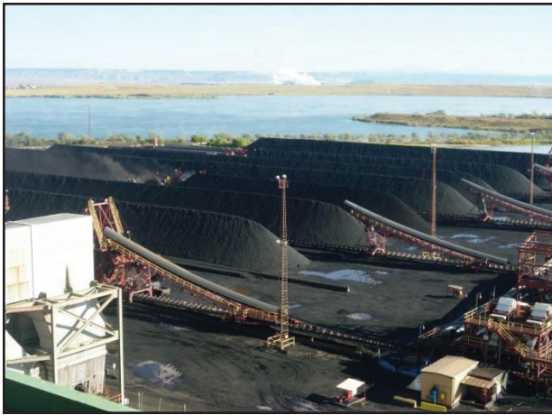
Coal preparation facility at FCPP, adjacent to Morgan Lake 164
